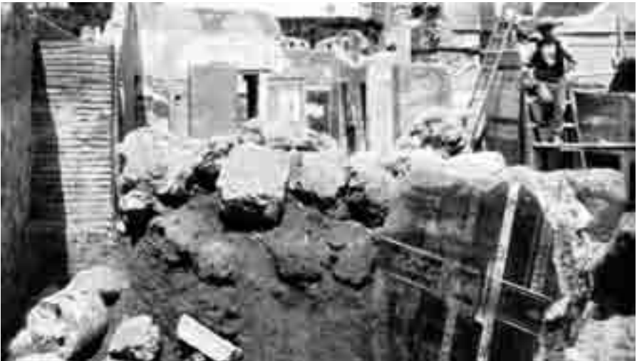
10. An excavation of the 1930s. Pompeian houses do not emerge from the ground in a pristine state. In fact, the force of the eruption means that they look rather as if they had been bombed. Here the painted plaster of the upper floor has collapsed into the rooms below.
